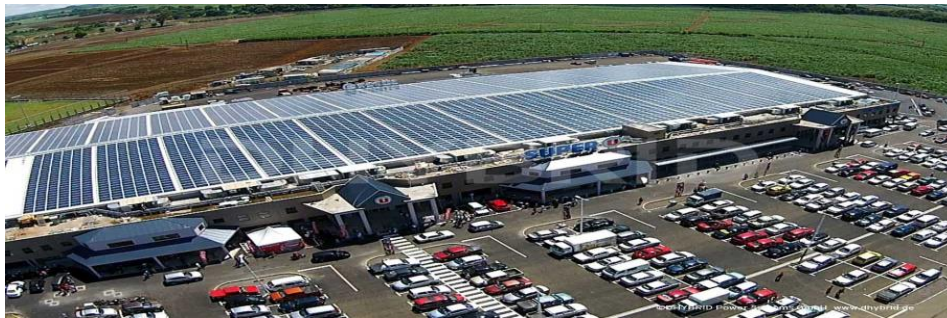
Solar panels at Super U Flacq
