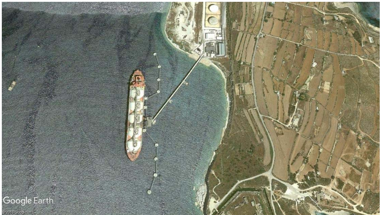
Figure 10-8 FSU based LNG Terminal, Delimara, Malta
